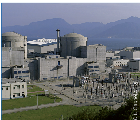
Class 1E Safety Equipment
