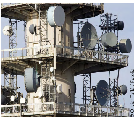
Telecom - Data infrastructure
